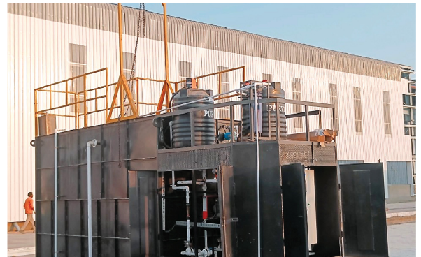
International Automotive Components, Pune (MBR, STP)
