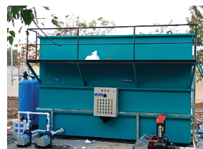
SBR (Sequential Batch Reactor)
