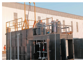
MBR (Membrane Bioreactor)
